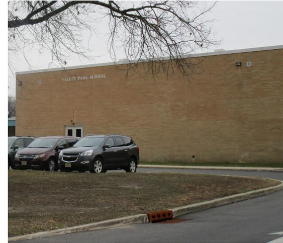
The two parking lots on both the east and west sides of the school can be converted to porous pavement to treat the stormwater runoff from the roof of the elementary school. A preliminary soil assessment suggests that more soil testing would be required before determining the soil's suitability for green infrastructure.
