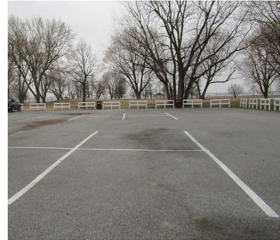
The basketball court can be replaced with porous asphalt which will also provide new asphalt for the basketball court. A rain garden can also be installed to the west of the parking lot to capture and treat stormwater runoff from the restroom building before it enters the catch basin. A preliminary soil assessment suggests that more soil testing would be required before determining the soil's suitability for green infrastructure.
